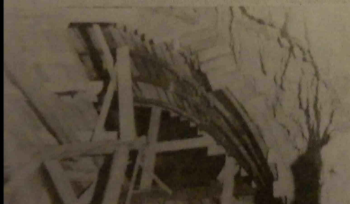
Graph No. 13 The beam supports arch rib which had to be cut small tunnels intersected a main tunnel.
